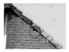
The gable brick ends shown exposed on the left have been fitted with bargeboards containing staircase type nest boxes. These will be faced with a plank with entrance holes cut for the Swifts to access the new nest places inside.
