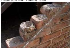
A Schwegler "Swift Brick" inserted into previously open eaves to provide a replacement Swift nesting place. The roof of this NHS hospital had to be sealed to meet hygiene requirements, but the Swifts' nests were saved.
