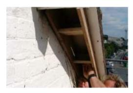
Plastic soffits and gutters have been fitted to this re-roofed house. Holes have been cut in the soffits close to the wall to provide access for the Swifts to their nests in the eaves.
