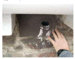
Swifts nest under the tiles on the brick ends of this roof. Repairs would evict them, but leaving the bricks as they are and fitting deeper tiles, offset to maintain the Swifts' access from below, will provide weather proofing and still let the Swifts nest.
